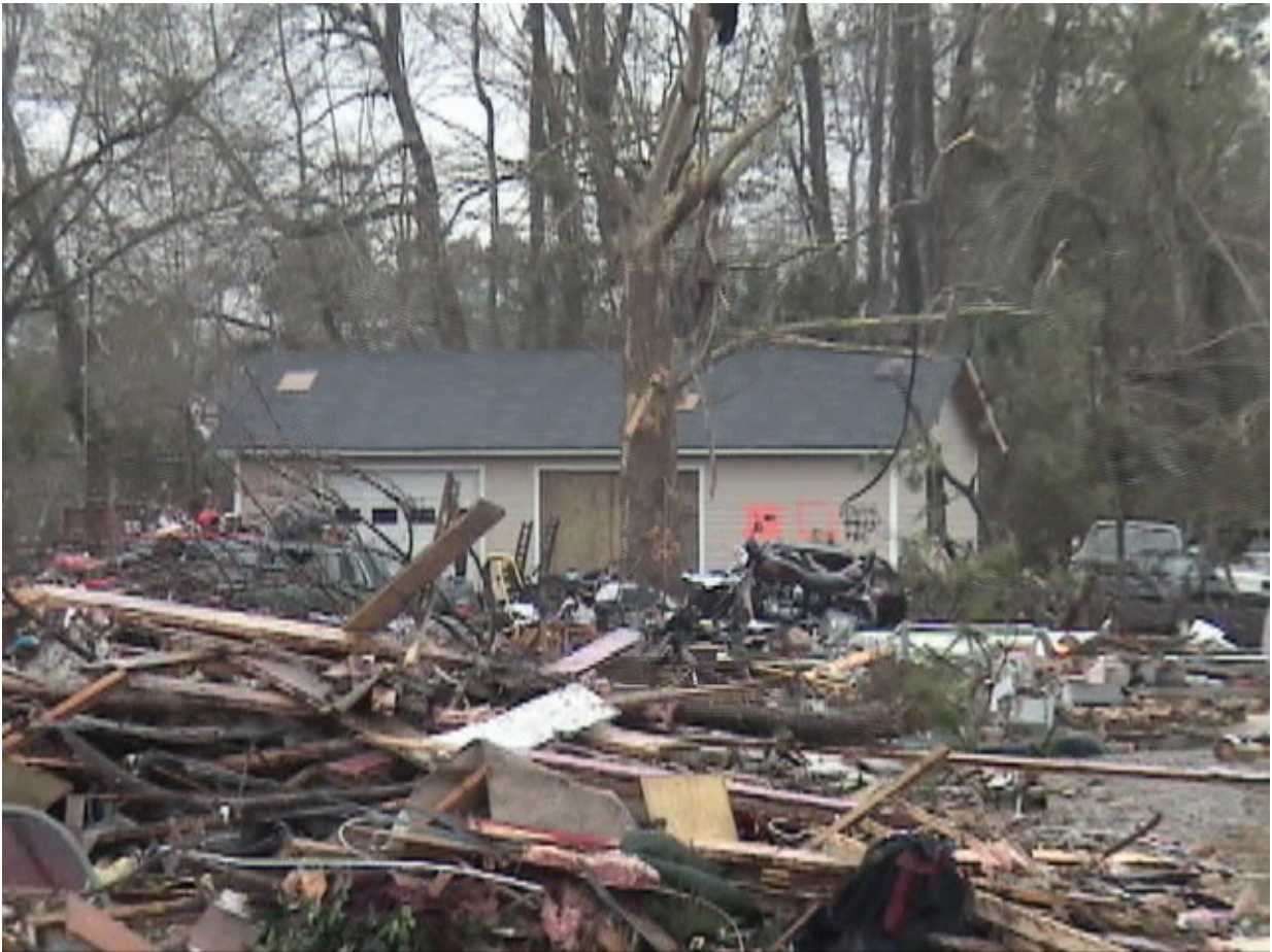
Figure 1. Tornado damage at Riegelwood, NC. Photograph taken by Cyn Johnson on 17 November 2006.
