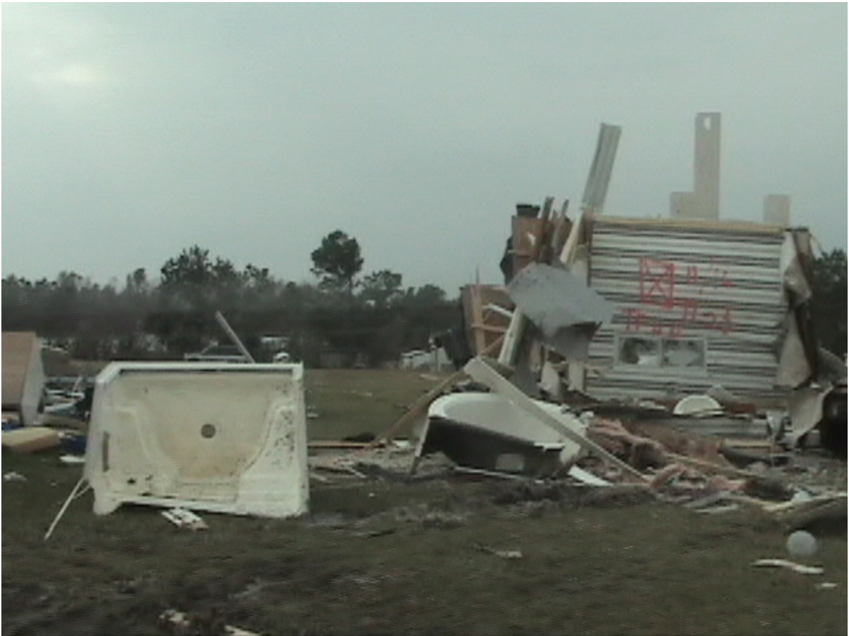
Figure 4. The remains of a shattered mobile home. Photograph taken by Cyn Johnson on 17 November 2006.
